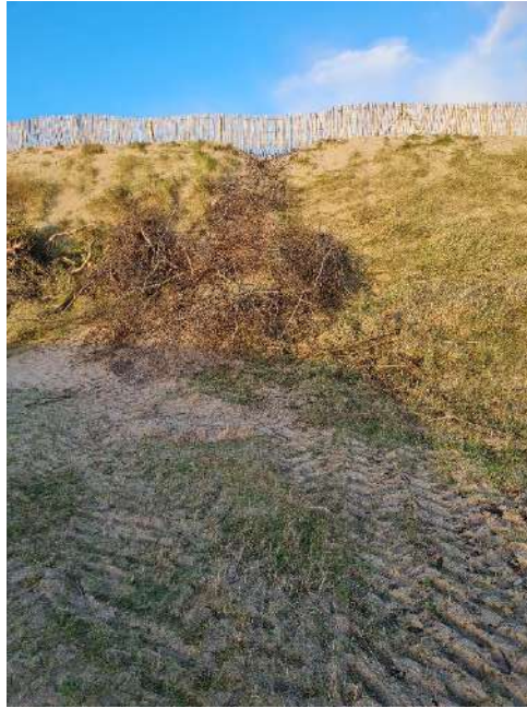
Figure 128 : Pose de branchages
